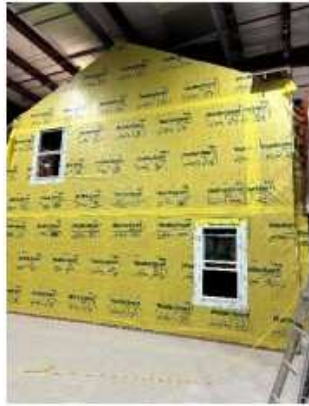
Mechanical-fastened WRB
