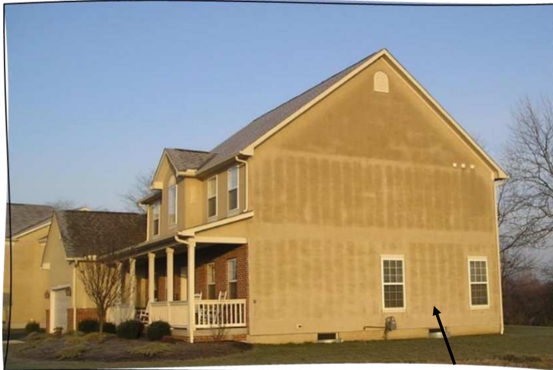
Conductive heat loss
